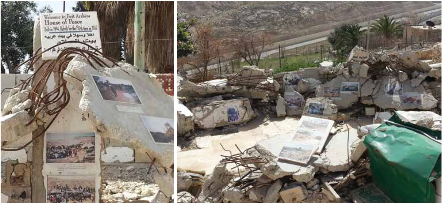
The Shawamreh home is now a peace center – Beit Arabiya- dedicated to the memory of Rachel Corrie and Nuha Sweidan, activists killed while protesting home demolitions © The Oakland Institute
