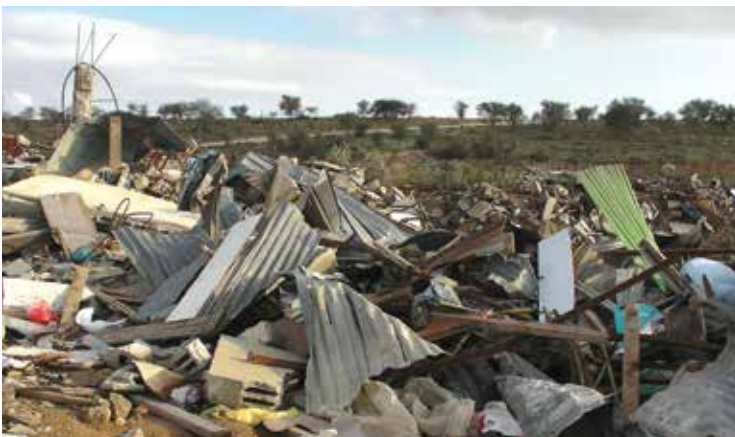
Rubble from the demolition carried out in January 2017 © The Oakland Institute
