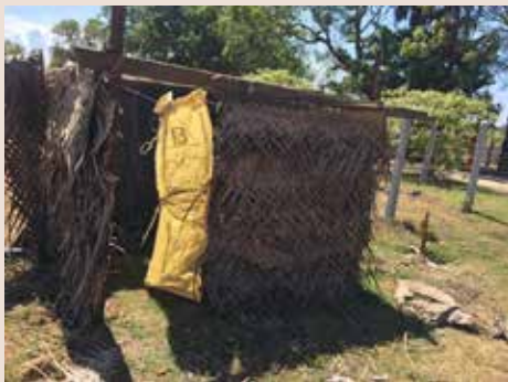
Toilet facilities for the resettled IDPs at Sampur
